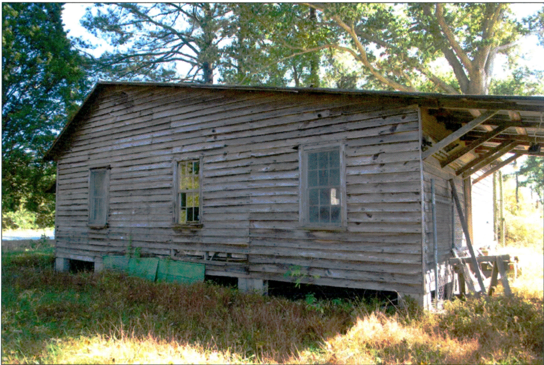
Tenant House (MT 1046, Property #46) Looking Southeast
