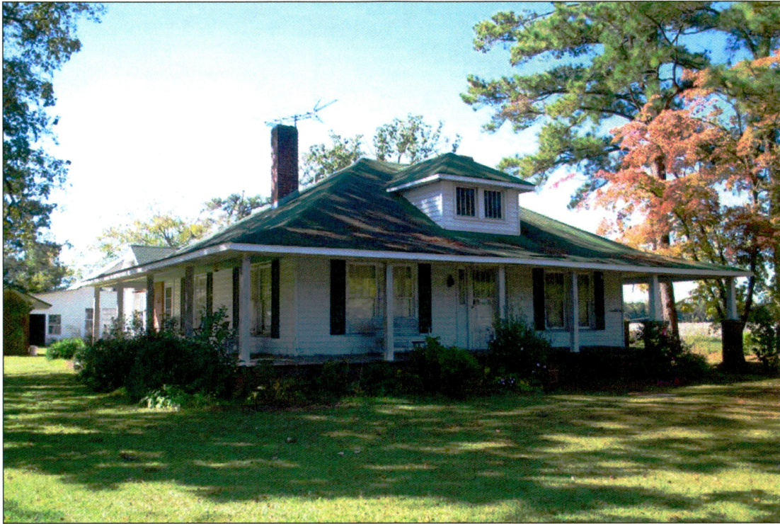
Jasper C. Griffin House (MT 1044, Property #45) Looking Northwest
